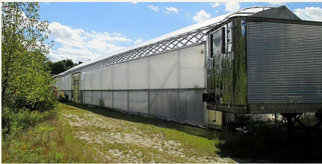
60 by 200 steel-frame greenhouse, ready to re-cover
